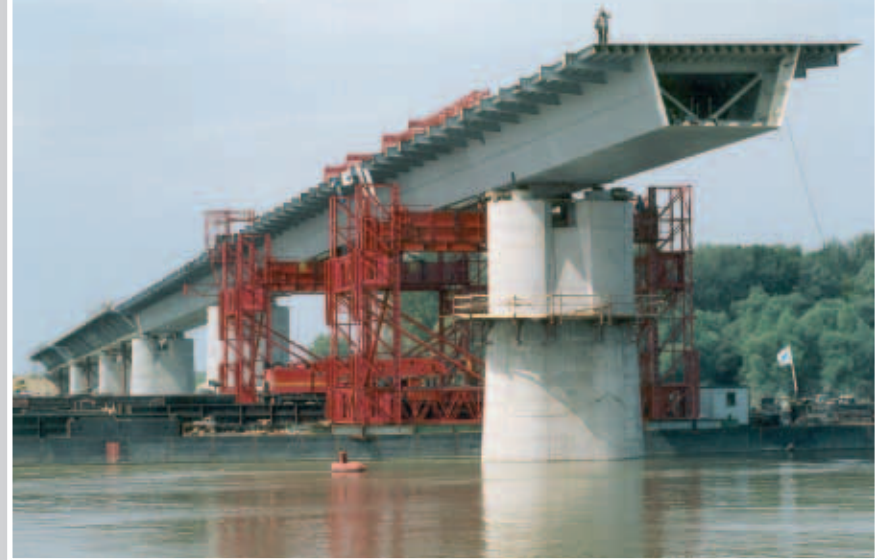
Constructing the main bridge
